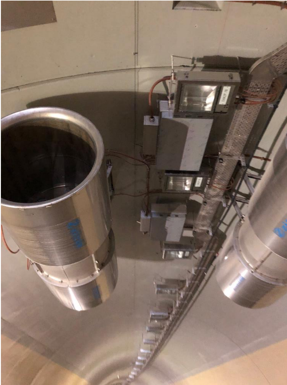
Figure 5. Jet fans with in-tunnel control units
